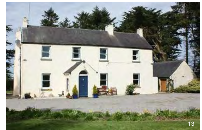
Simple matching openings across the entire facade complete with a porch of the same finish. Dunlavin, County Wicklow.
