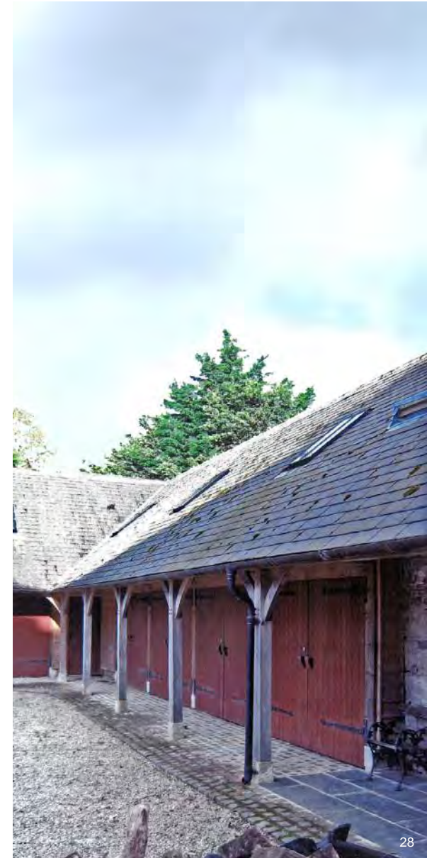
Dutch barn outbuilding conversion. County Wicklow.
